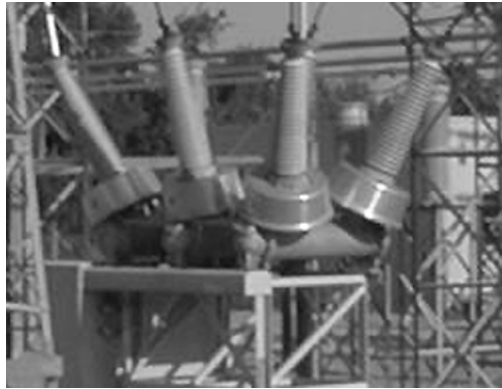
FIGURE 2.6.28 High-voltage circuit breaker with BCTs mounted underneath a metallic cover. (Photo courtesy of Kuhlman Electric Corp.)
