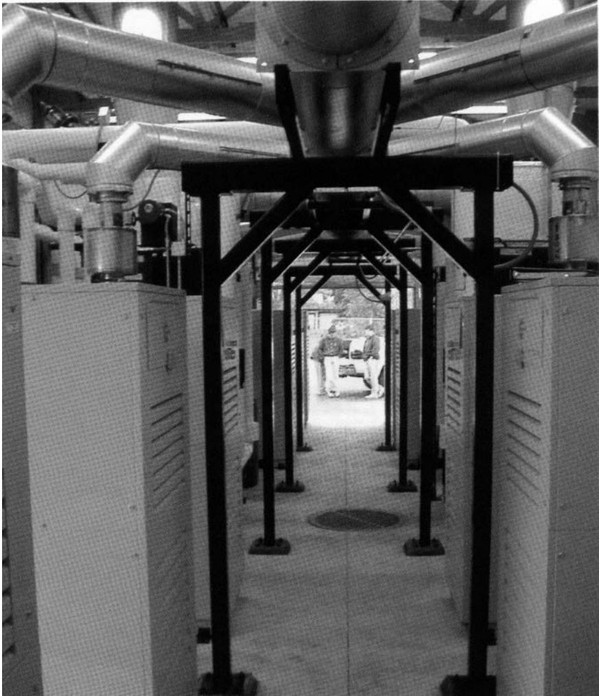
Figure 17-5. Installed Microturbines.
