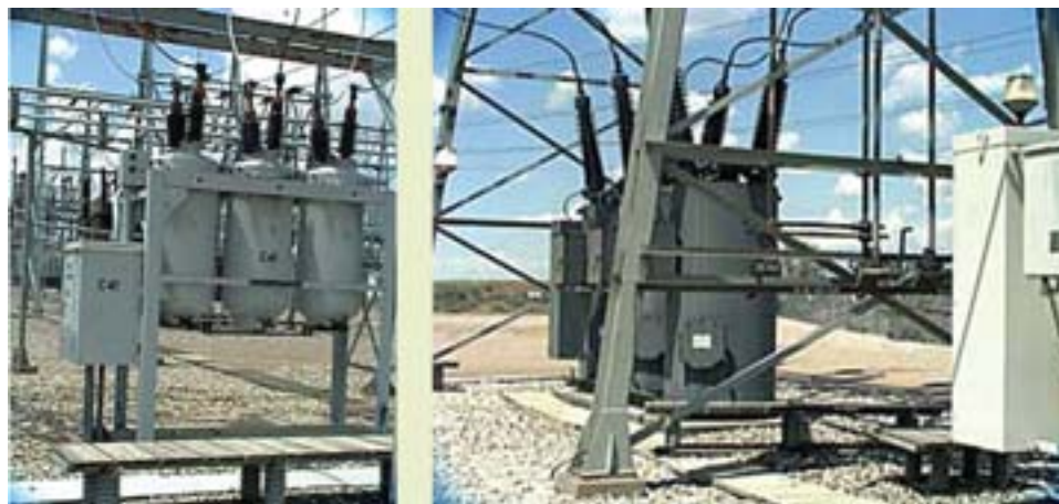
Oil Circuit Breakers
