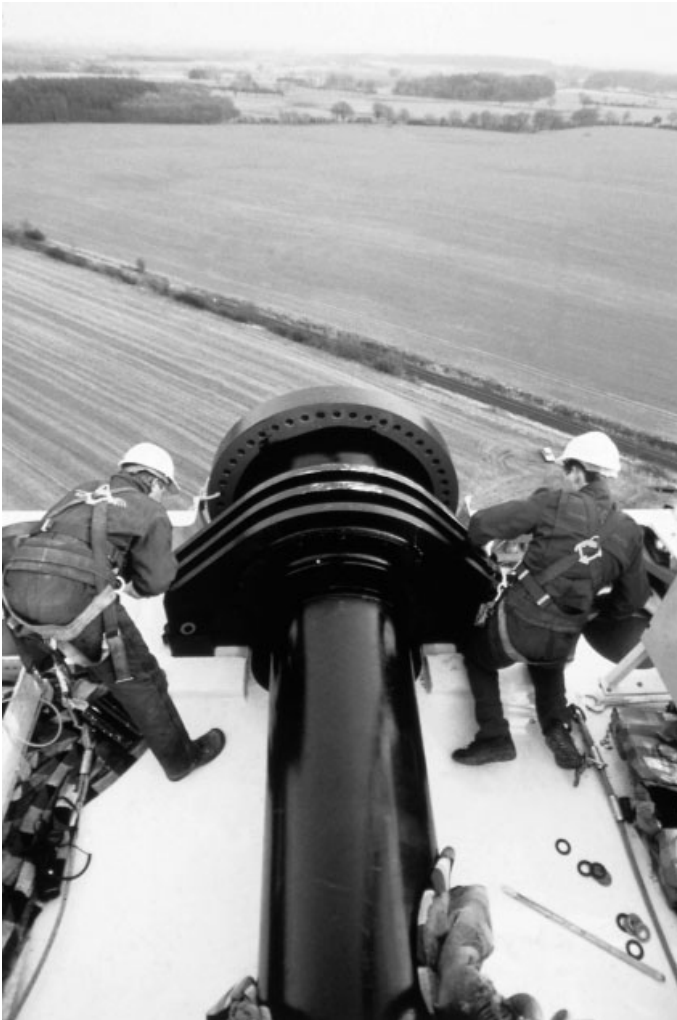
Figure 6.19 Turbine Assembly in the Air (2). (View of low-speed shaft and front bearing after installation on 1.5 MW NEG Micon turbine). (Reproduced by permission of NEG Micon)
